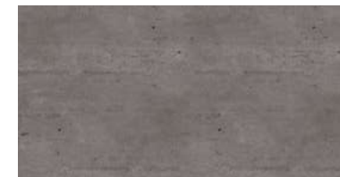
10 BETON BETON BETON BETON
